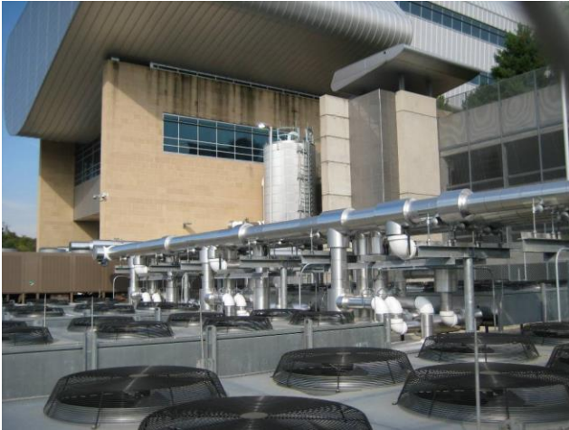
Figure 3. Dry Coolers/Chillers
