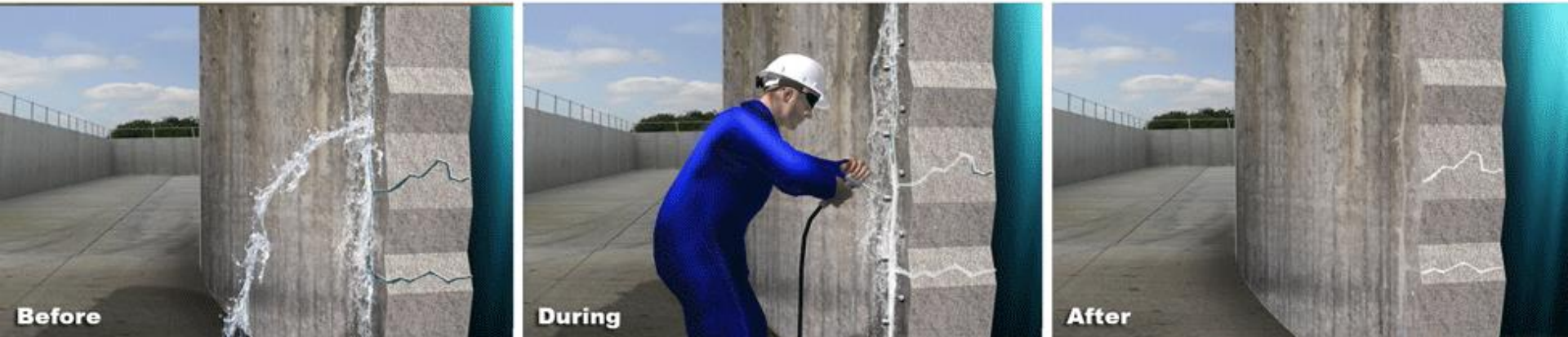
Crack Injection
