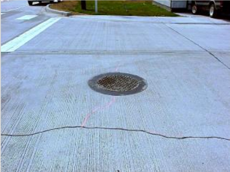
Cracking
