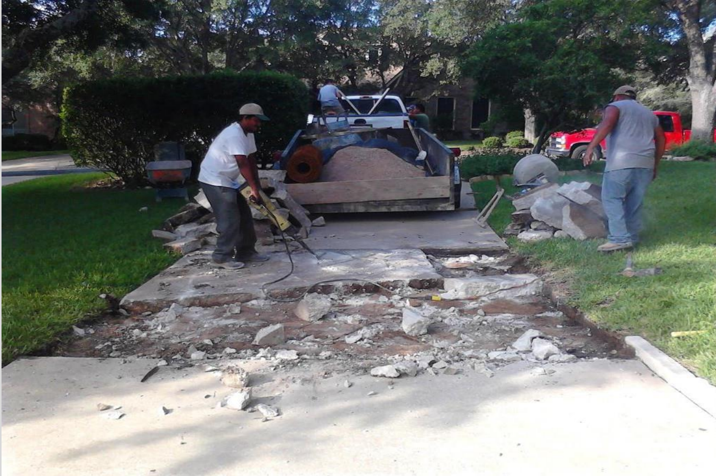
Tear Out & Replace
